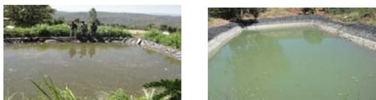
Figure 4. Trapezoidal pond covered with pvc plastic in study area
